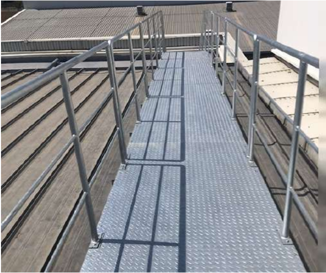
PLATFORM ON ROOF
