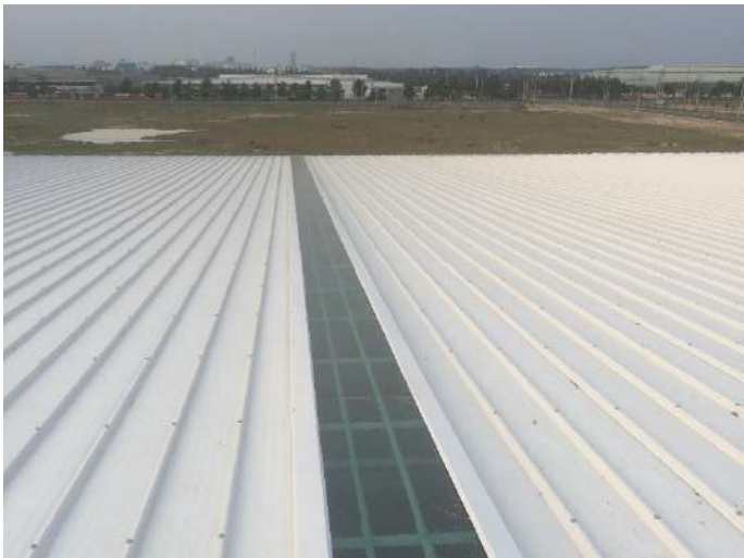
TEMPERED GLASS ON ROOF
