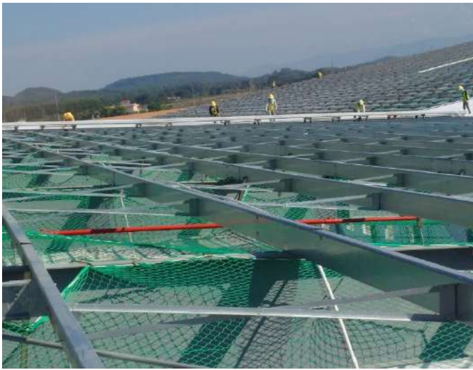
PURLIN BRACING - SAG ANGLE
