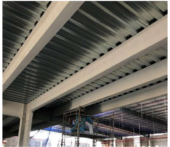
FIRE PROOFING PAINT
